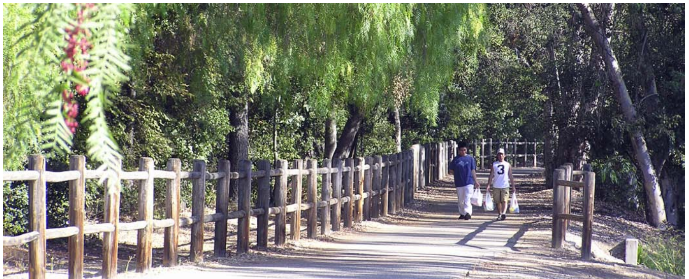
Ojai Valley Trail, California — A 5-mile extension to this charming 10-mile trail was railbanked in June 1996. Parallel asphalt and dirt tracks accommodate walkers, bicyclists, inline skaters and equestrians.
