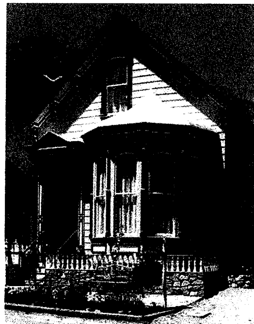
58 B Street, Virginia City, Nevada (1875). Rehabilitated as a bed and breakfast. Courtesy Chris Echin.
