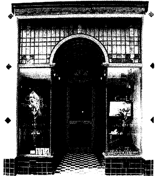
114 NW Main Street, Rocky Mount, North Carolina (1928). Photograph: William Ferguson
